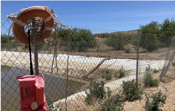
A basin filled with groundwater was used to mix cement for the border wall under construction during President Trump's first term. This photo was taken in 2021, soon after he left office. (Peter O'Dowd/Here & Now)
